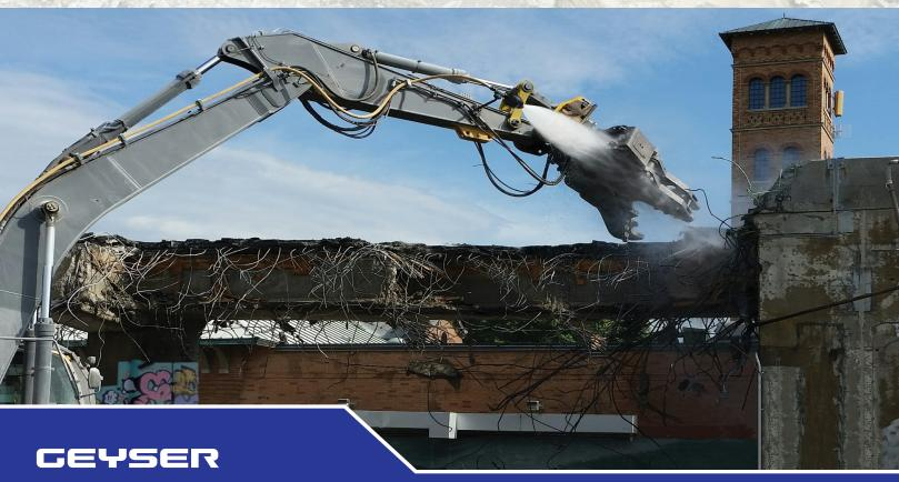
The GEYSER is designed for complete ultra-high reach dust control. The GEYSER installation best operates together with the pump of any V-500 series dust control machine. The GEYSER atomizing nozzle is mounted on the stick of an excavator, catching airborne dust at the source. As material falls to the ground, ensuing dust particles are captured by the V-500 water cannon aimed at the landing zone.
